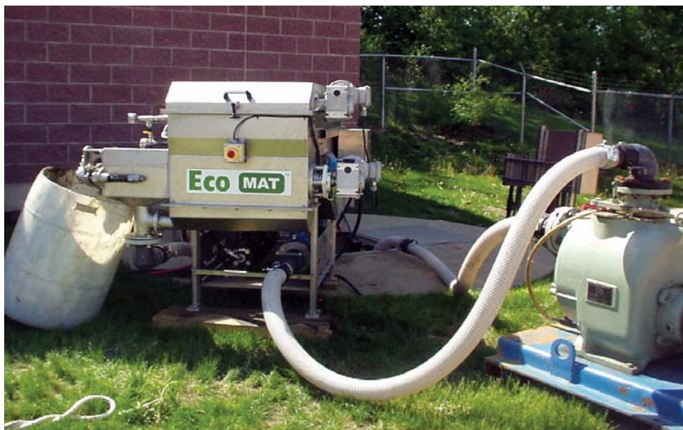
Figure 6. 0.5 mgd Capable Unit Tested at City of McHenry Wastewater Treatment Plant
